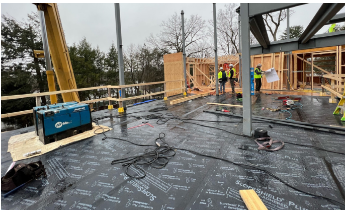
Durable to foot traffic and heavy equipment, SlopeShield Plus SA can withstand 6 months UV and climate exposure. Installation College Building, Amherst, MA
