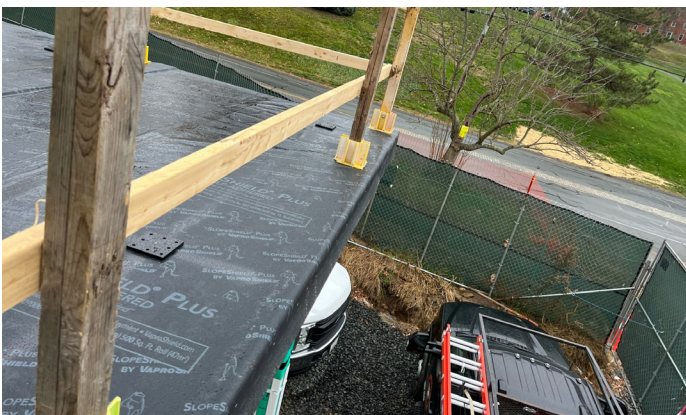
End grains are especially susceptible to water intrusion. By allowing SlopeShield Plus SA to overhang the structure, end grains are protected when water is squeegeed from the deck after and during rain events. Installation: College Building, Amherst, MA
