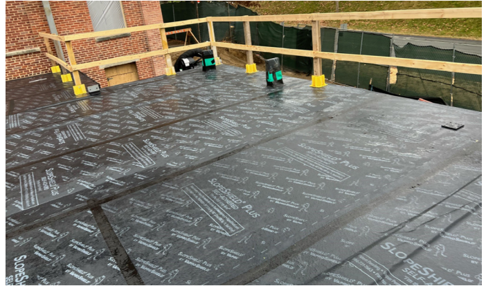
SlopeShield Plus SA installed with VaproTape will protect the mass timber floor or deck from bulk water infiltration. Installation College Building, Amherst, MA
