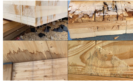
Outer portions of mass timber layers may dry disproportionately faster compared to the inner layers, causing checking, staining, dimensional changes, and compromising structural values.
